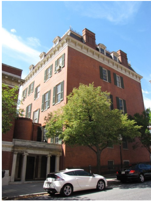
View of the rear (south) and east elevations.
